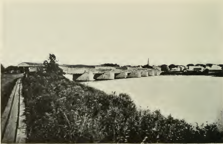
Bridge Connecting Schenectady and Scotia, 1809 to 1873.
